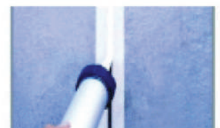
Step 2: Fill the gap with VIVA Flex.
