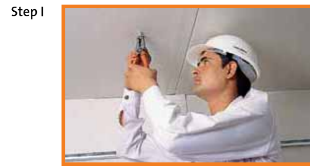
Rawl Plug fixed into the soffit
