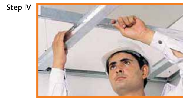
Intermediate channel and ceiling section are connected with each other by using connecting clip
