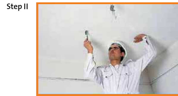
Rawl Plug with soffit cleat is fixed into the soffit
