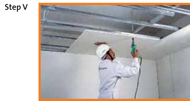
Plasterboard screw fixed with Drywall screws in staggered joint manner
