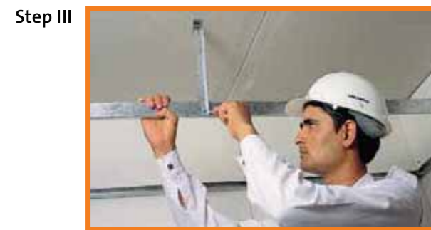
Intermediate channel connected to ceiling angle at required suspension height
