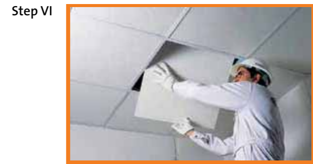
Ceiling panels are laid on the grid
