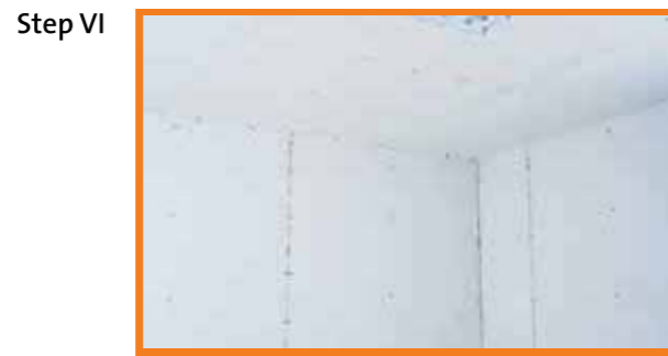
Plasterboard fixing complete, ready for jointing & finishing
