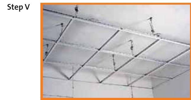
Completed framework with "T" section, ready for laying ceiling panels
