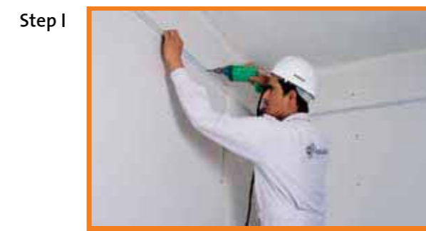
Wall angle fixed to the perimeter of the wall at the ceiling level
