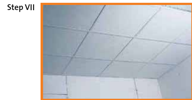
Finished grid ceiling
