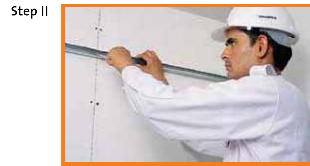
Perimeter channel fixed to the wall at required ceiling
