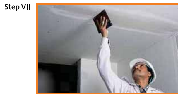
Jointing & finishing is done on tapered edge/square edge joint
